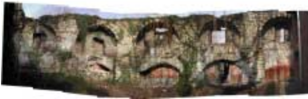
Fig 6. Global overview of the critical part A – city side
