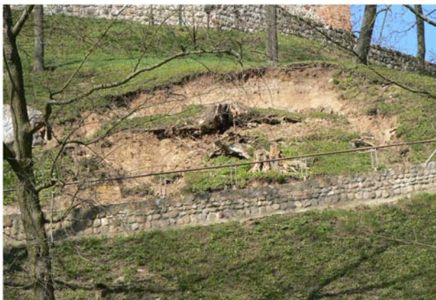
Fig. 3. Slip of the Gediminas mound slope (Photo by Vaitiekūnas)
