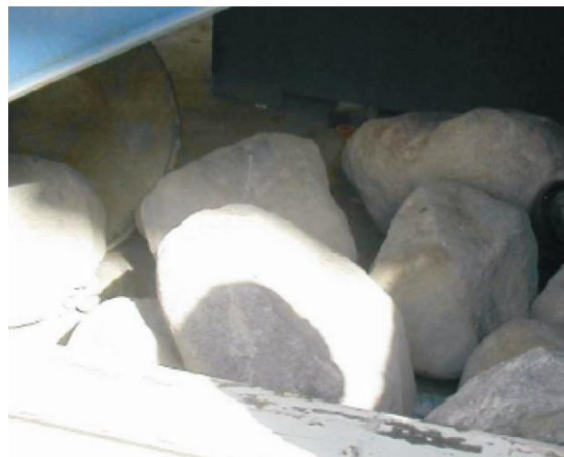
Fig. 6. Some boulders given during TURL1 mechanized excavation
