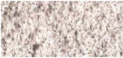
Fig. 8. Macro structure of plaster without lightweight aggregate
