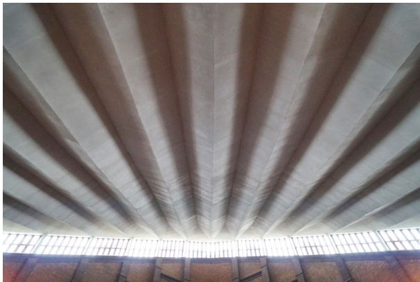
Figure 9. View of the accordion-like structure of the ceiling
